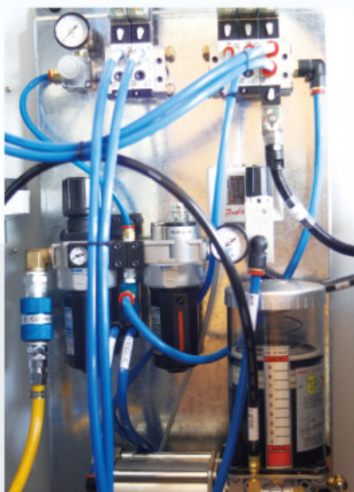
Lubrication and Pressure System
